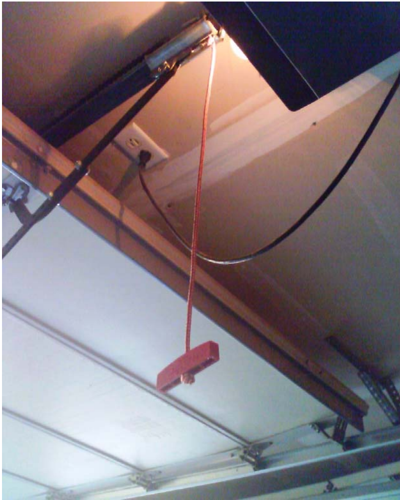
The garage door release rope. Pull to release the door, but only if you're sure it won't cause the door to slam closed
