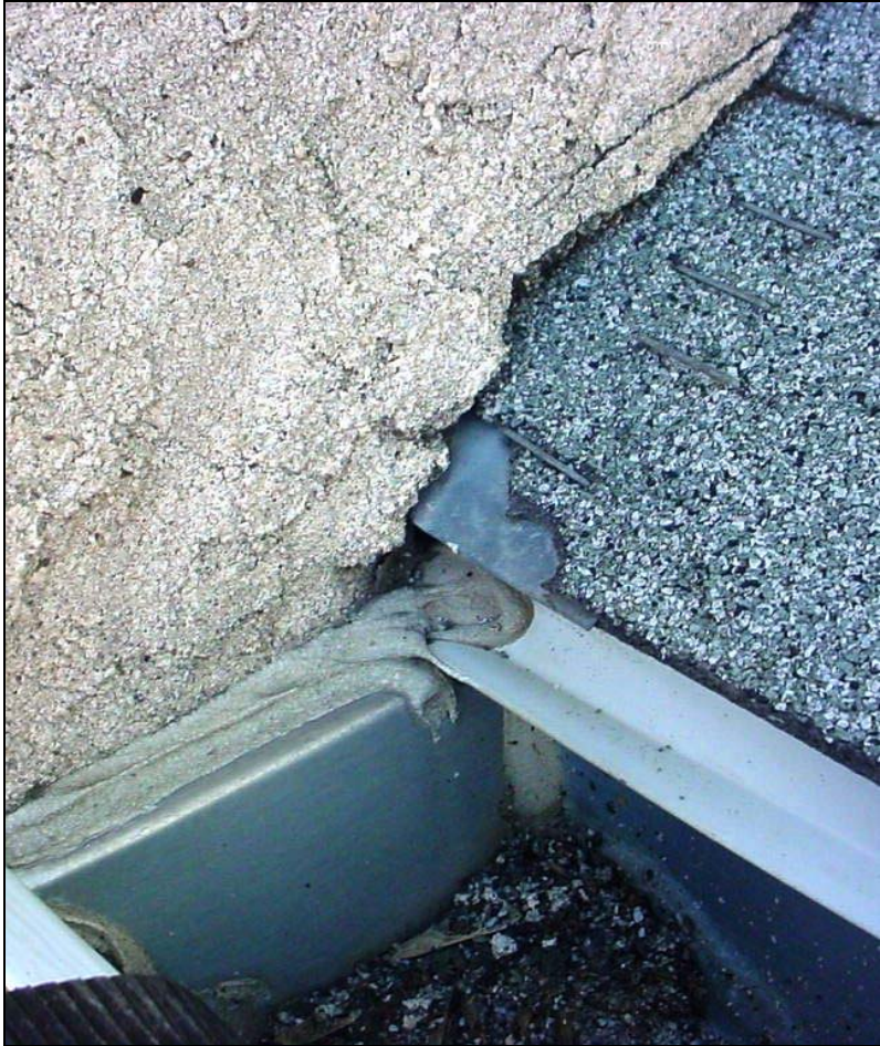
Interface between stucco, asphalt shingle and rain gutter
