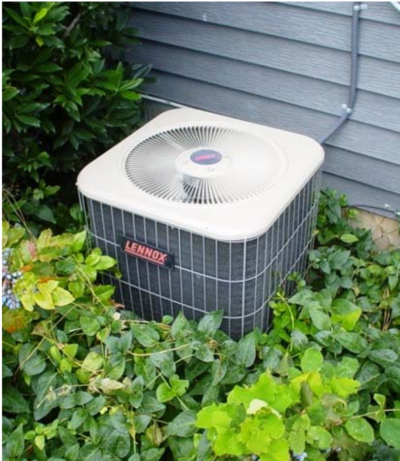
The central air compressor must be kept free of dust and weeds
