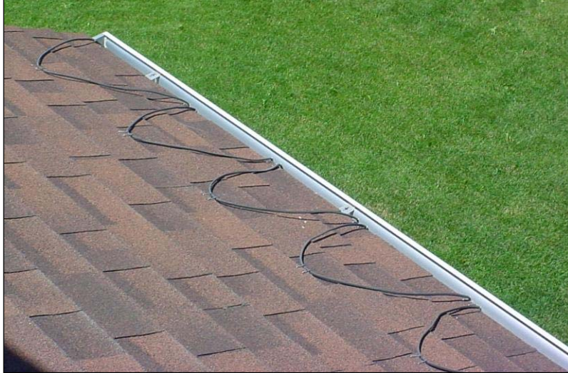
Heat tape used near the drip line to discourage ice damming
